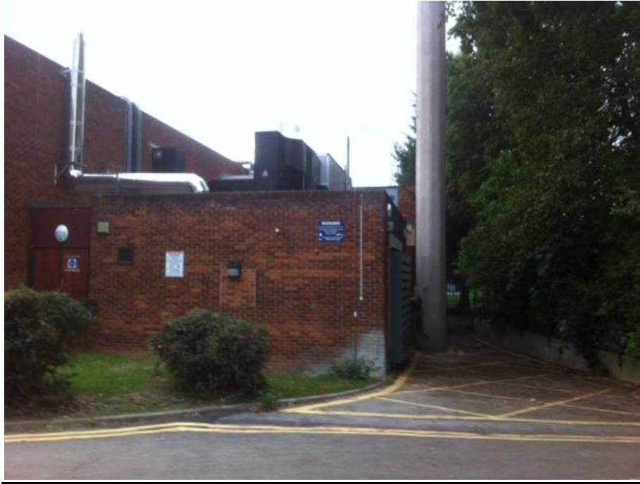
Location of boiler flue
